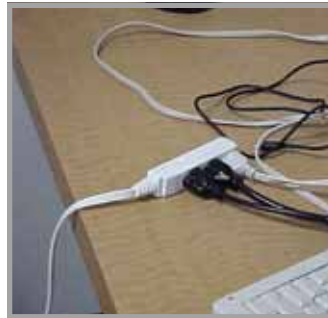
Extension cord used as a substitute for permanent wiring
